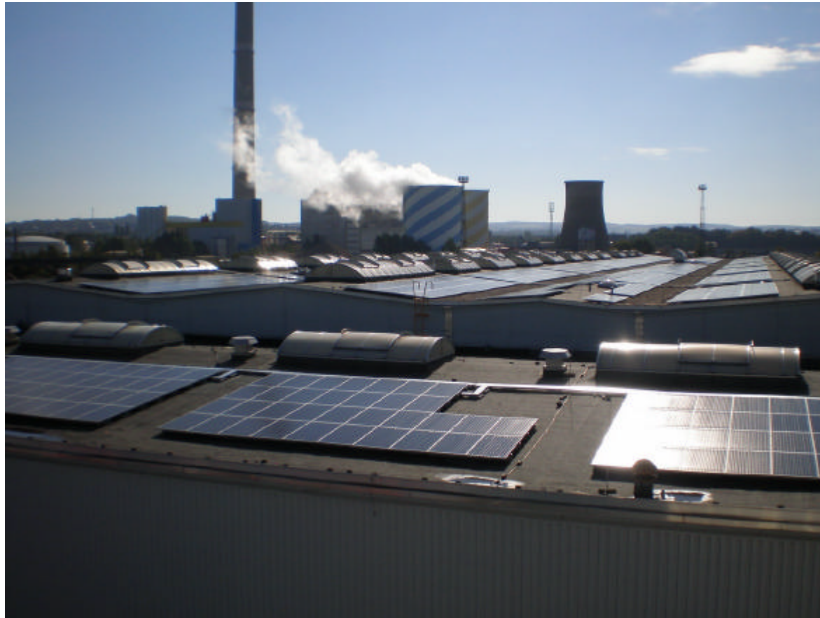
view: module array – flat roof
